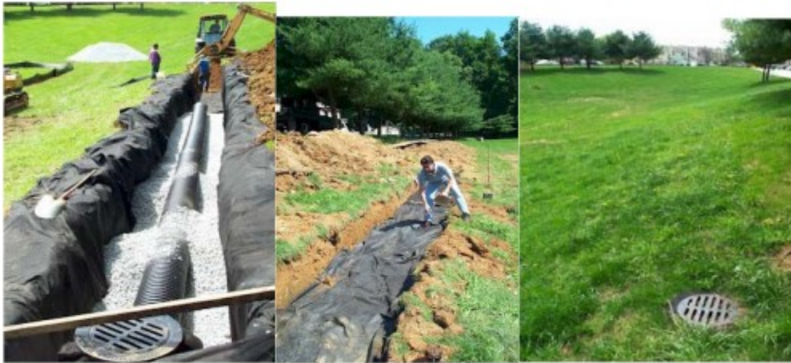
Figure 4: Example of Infiltration Trench Installation
