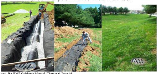
Figure 4: Example of Infiltration Trench Installation
