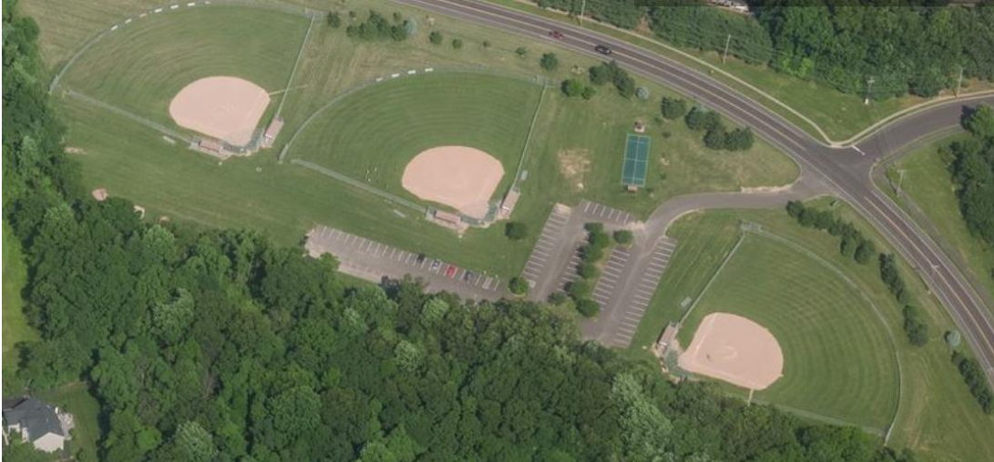
Building 1 – Fred Allan Softball Complex Concession Stand, Restrooms, Pavilion
