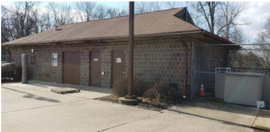
Building Number 3 – Pool Bathrooms at Lap Pool – Constructed in 1995
