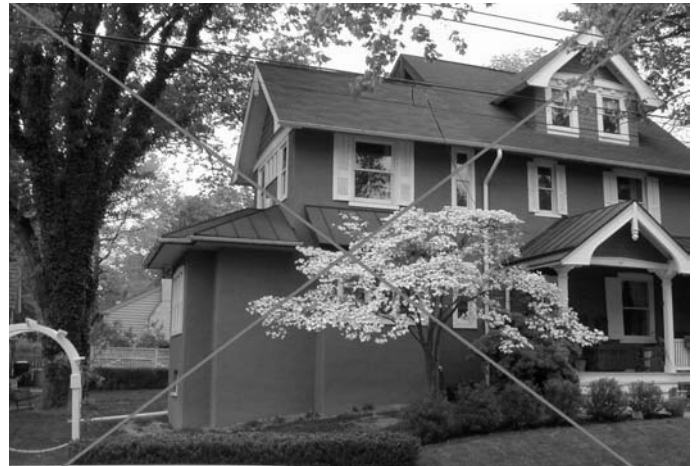
Illustration 36: Inappropriate addition due to a lack of offset between the original and the addition, and the mimicry of window details
