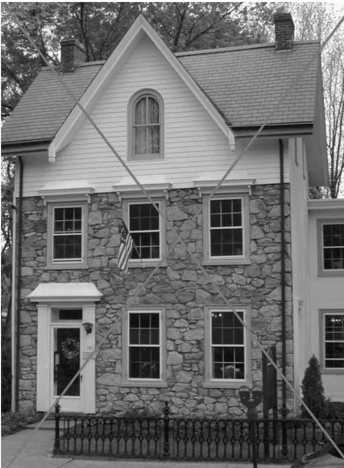
Illustration 34: Inappropriate addition due to the removal of the original stucco and the raising of this two story building to add a third floor
