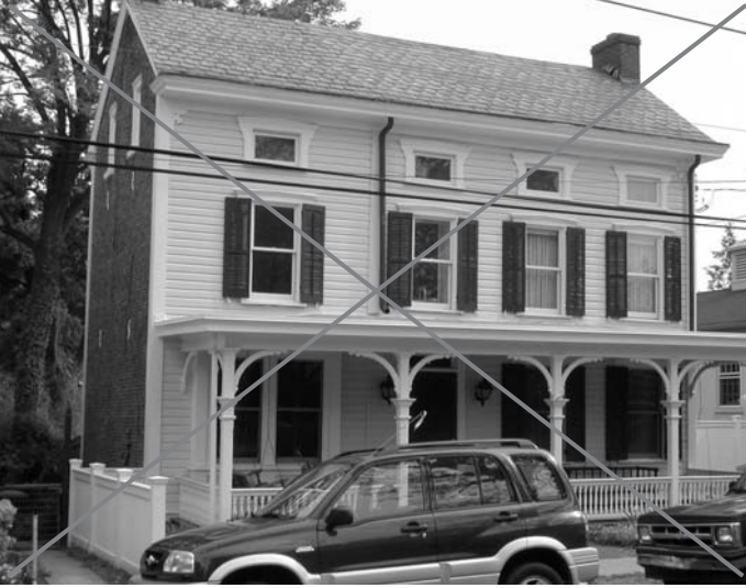
Illustration 33: Inappropriate addition due to the mimicry of clapboard, window details and the lack of a recessed wall plane
