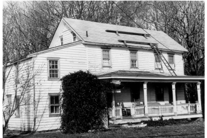
Illustration 3: Work in progress at Bennett house
