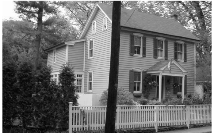
Illustration 27: Appropriate clapboard addition for its change of roofline, similar materials, wall plane and avoidance of copying windows.
