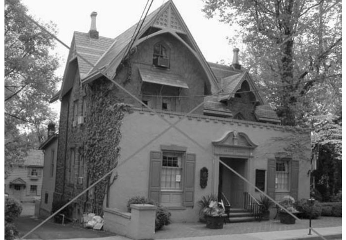
Illustration 35: Inappropriate addition due to the concealment of the original Victorian era structure with a colonial type front facade
