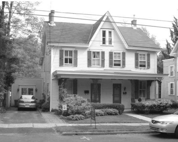
Illustration 32: Appropriate side yard addition for its recessed wall plane and similar clapboard and trim details
