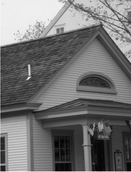
Illustration 41: Appropriate infill due to its clapboard dimension, porch detailing, and window and roof details
