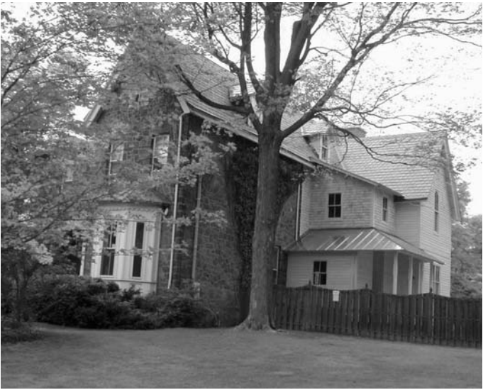
Illustration 31: Appropriate shingle and clapboard addition to this stone structure for its changes of material and roof lines
