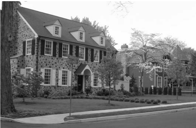
Illustration 43: Appropriate infill due to the window proportions and details, dormer proportions, front yard setback and traditional stonework
