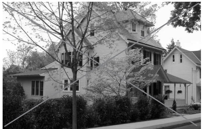
Illustration 37: Inappropriate addition due to the use of casement windows and low pitched roof
