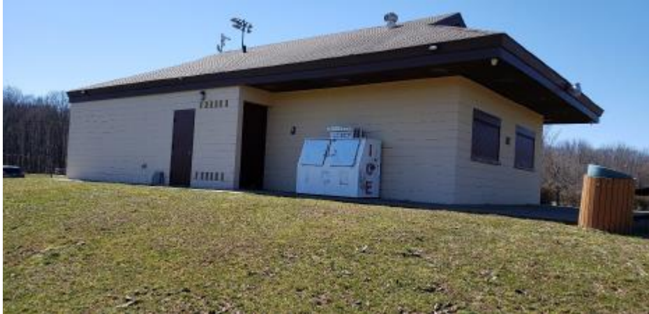
Building 1 – Restrooms and Concession Stand
