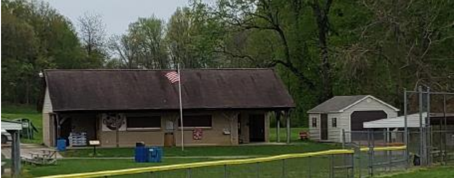
Building 2 – Robert Stoddart Fields Concession Stand, Restrooms, Pavilion – Edgewood Road
