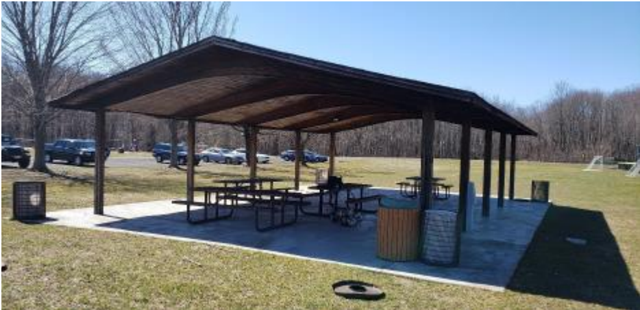
Pavilion at Fields C & D
