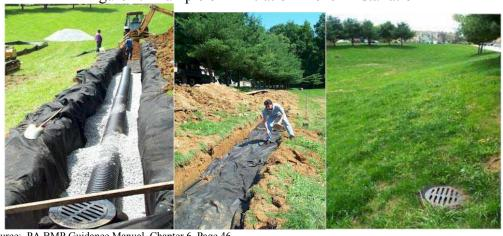
Figure 4: Example of Infiltration Trench Installation
