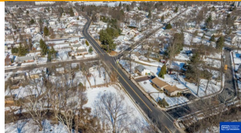
East Hancock Street Rehabilitation, Lansdale Borough, PA
