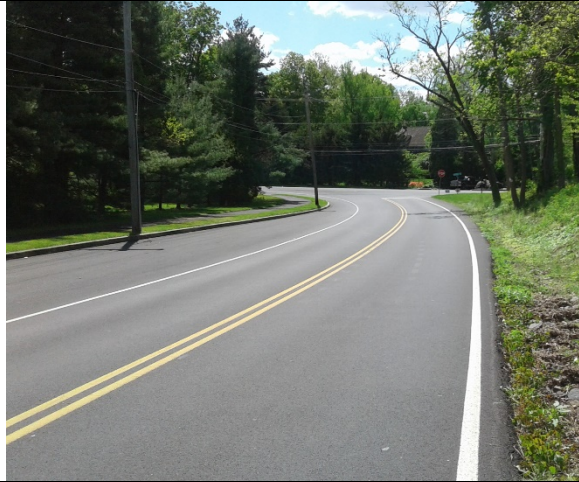
Dolington Road shoulder toward Quarry Road Intersection
