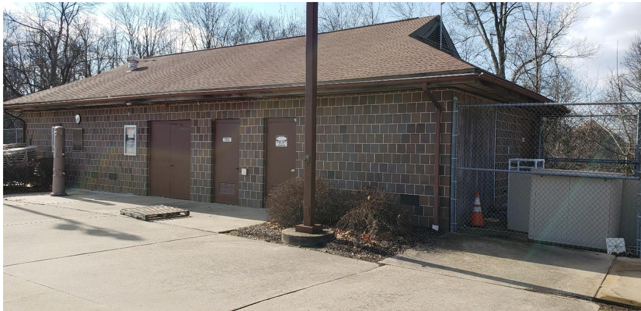
Building Number 7 – Pool Bathrooms at Lap Pool – Constructed in 1995
