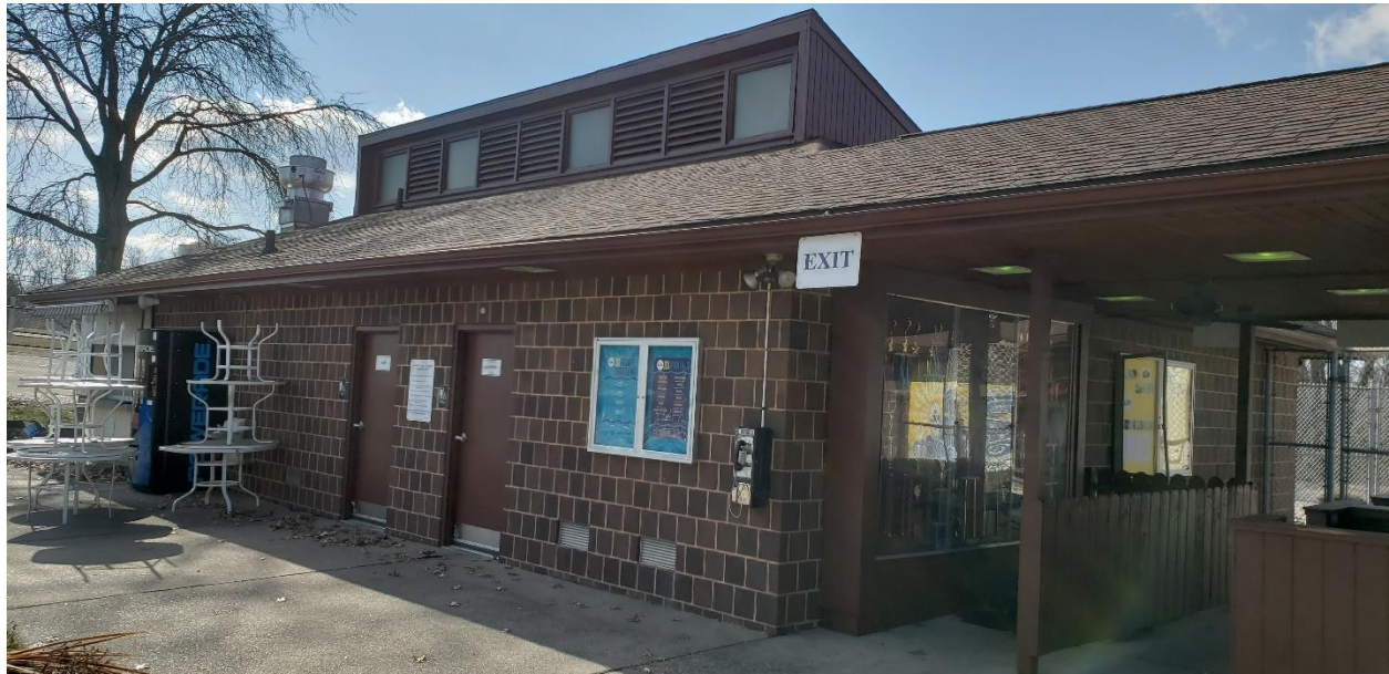
Building Number 6 – Pool Bathrooms & Snack Bar – Constructed in 1981
