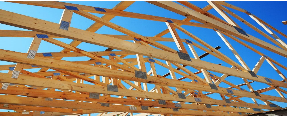
Example of roof truss construction (this will be scene in the attic or ceiling of top floor)
