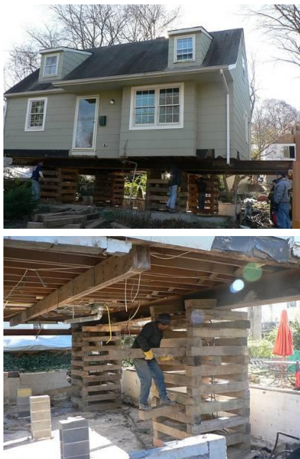
Figure 6.1-2 Yardley Borough Elevation Project
